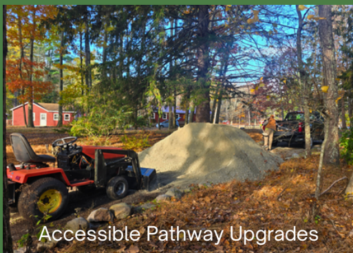
Accessible Pathway Upgrades
